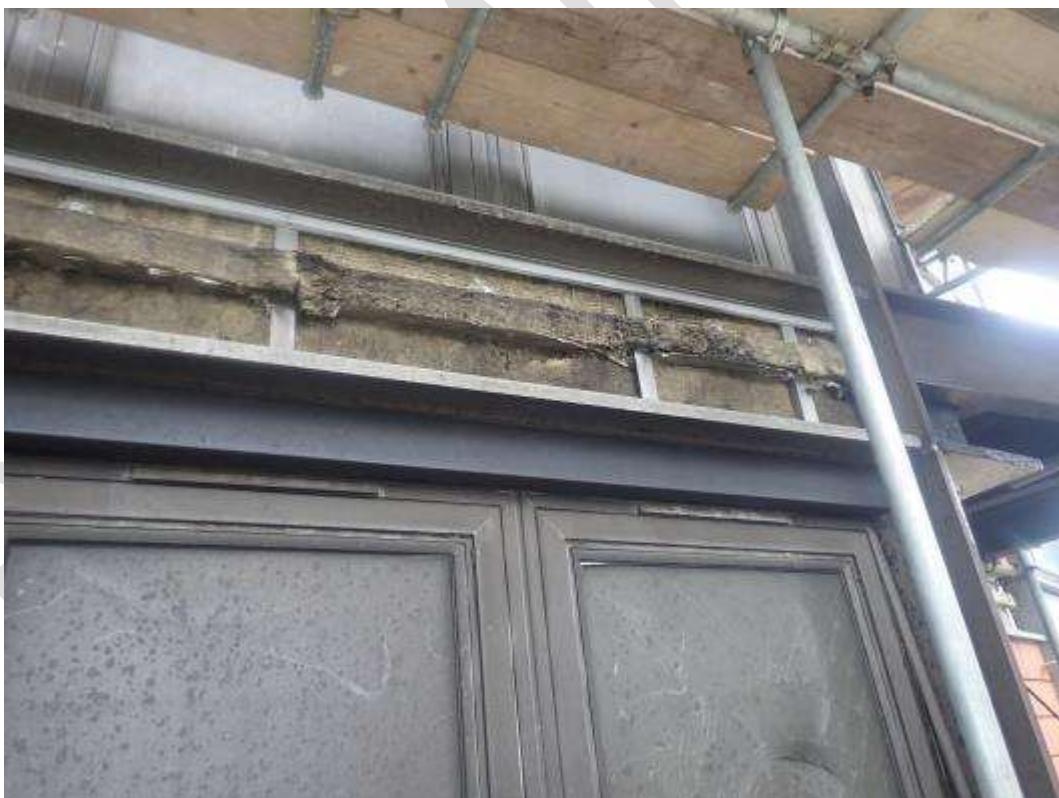
Image showing the internal construction of the ACM cladding between the 9 th and 10 th floors
