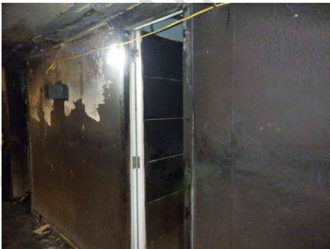
Image showing the AOV door on the 8 th floor
