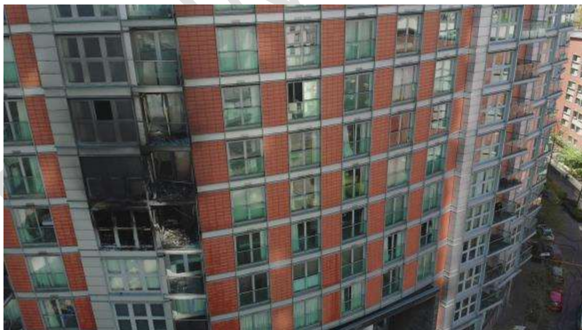
Images showing the damage to the exterior North face of NPW
