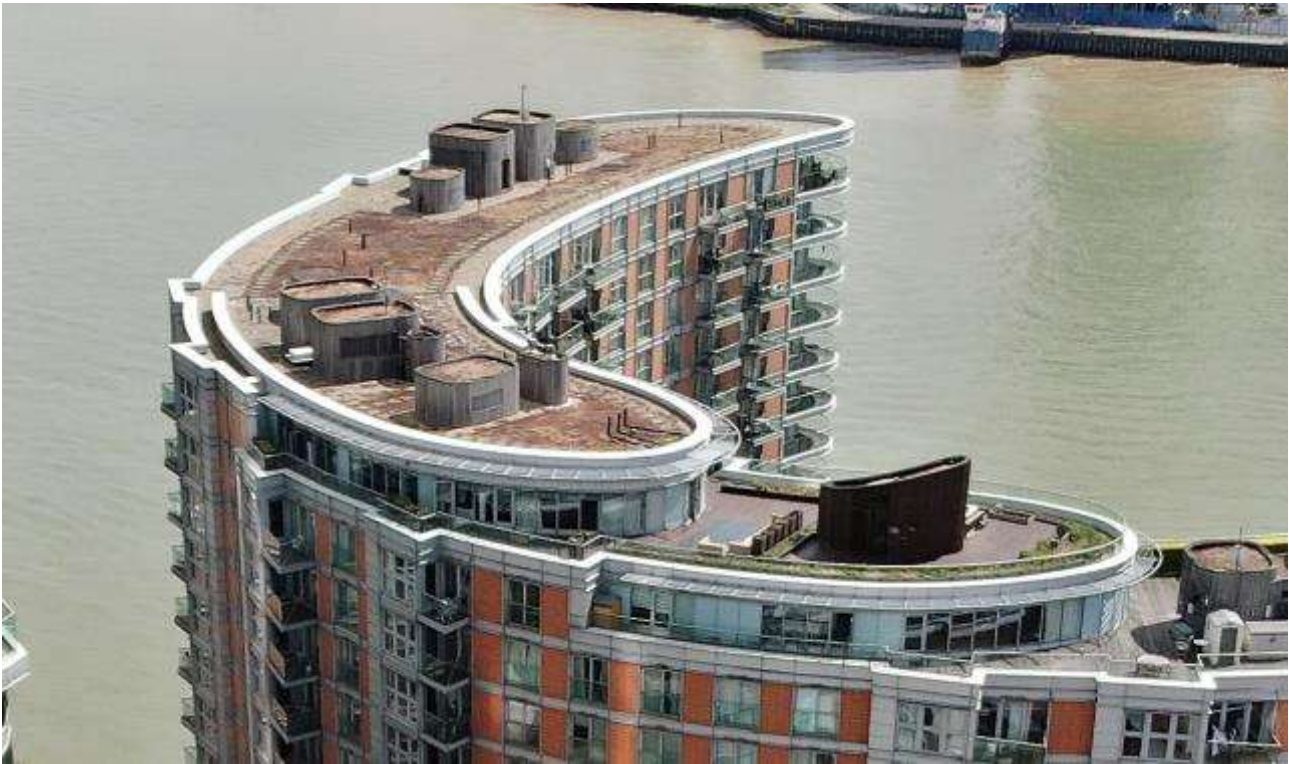
Image showing the roof of NPW with AOV vents
