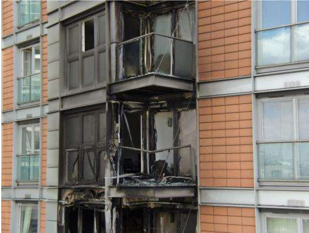
Image showing the external fire damage on the 9 th and 10 th floors
