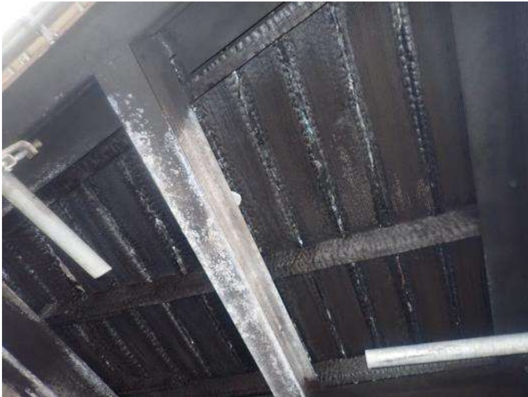
Image showing the charring to the underside of the 9 th floor balcony timber decking
