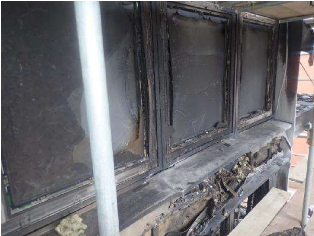
Image showing the damage to the ACM cladding between the 8 th and 9 th floor windows
