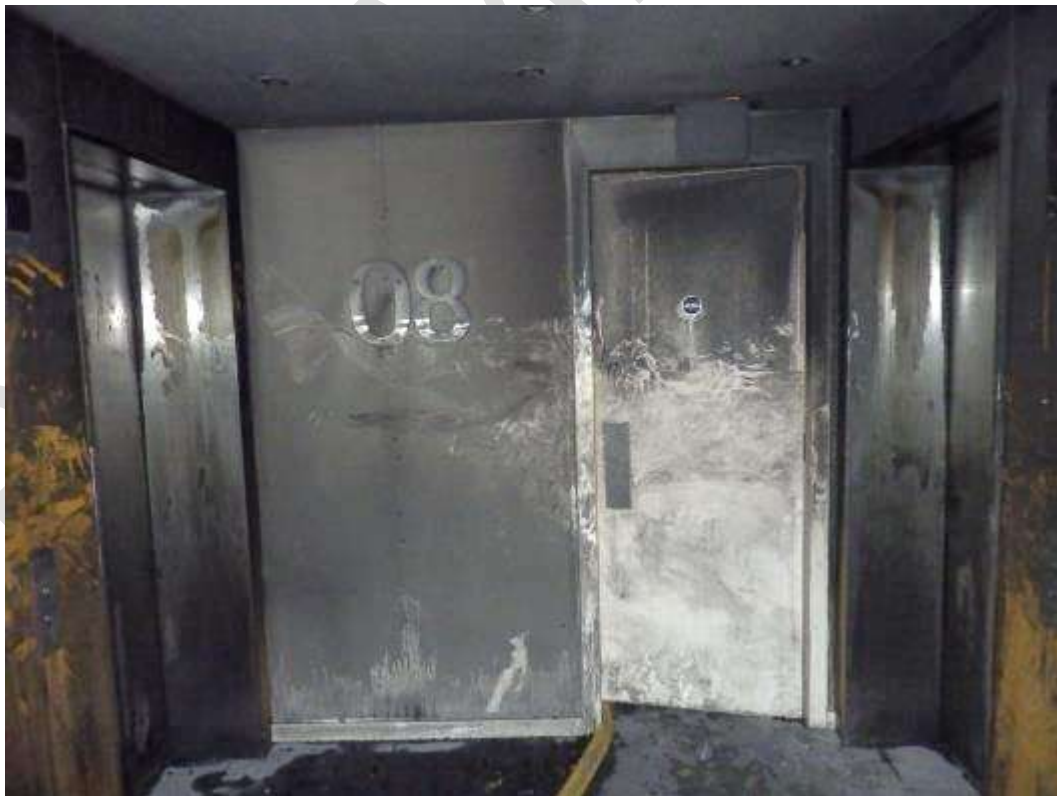
Images showing the external and internal view of the door at the head of the 8 th floor stairwell
